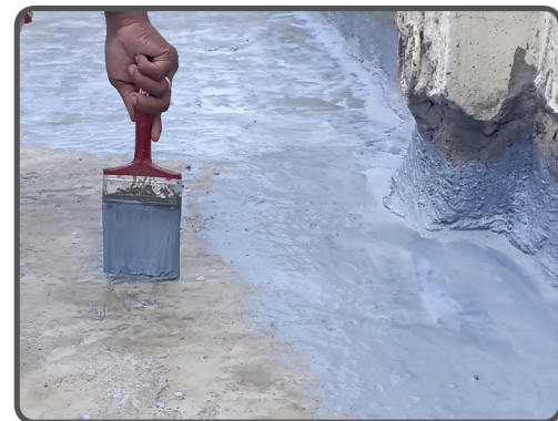
Apply to Surface 1st Coat Vertically & 2nd Coat Horizontally
