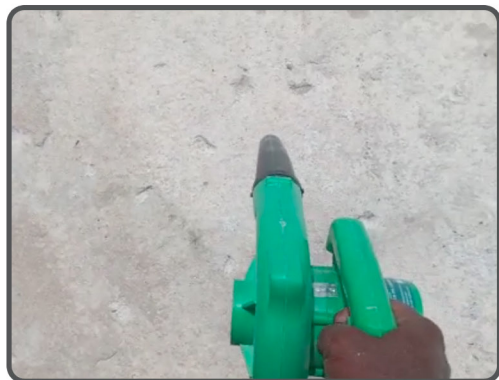
Clean the surface, removing dust, & oil, grease, and loose particles
