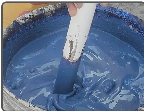
Mixing water proof oil & Portland Cement 1:1 Ratio
